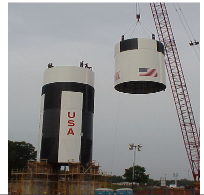
Penwal oversaw installation of the replica in record time.
